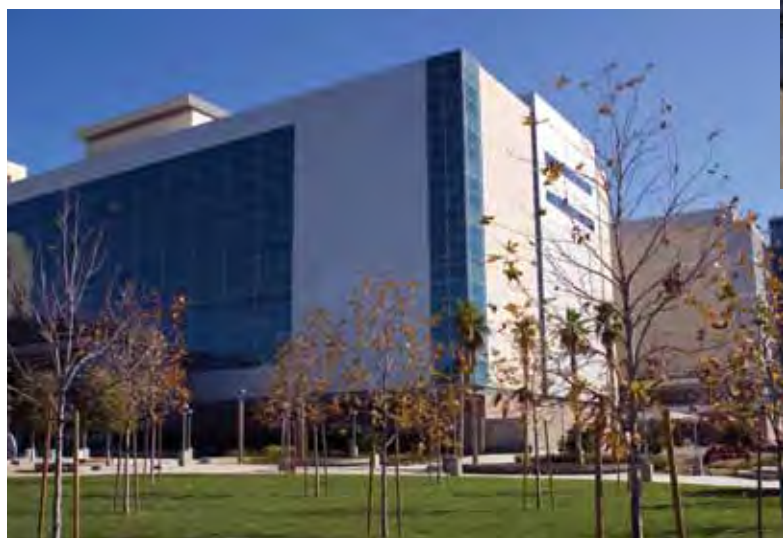
The 1.5 million-square-foot Los Angeles County + USC replacement facilities have opened nearly 15 years after the 1994 Northridge earthquake rocked Southern California. The project cost $1.02 billion for construction and equipment.
